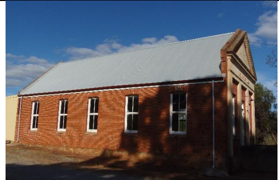
West façade Source: Stephen Carrick Architects October 2021
