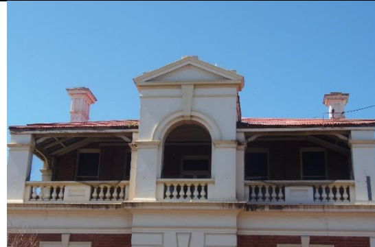
Central bay with pediment Source: Stephen Carrick Architects September 2021
