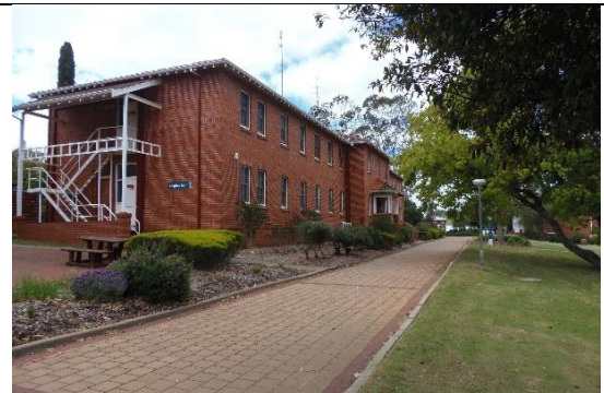
Hughes Hall to the east of Dempster Homestead Source: Stephen Carrick Architects October 2021
