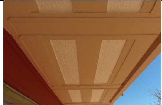
Pressed tin ceiling to awning Source: Stephen Carrick Architects September 2021
