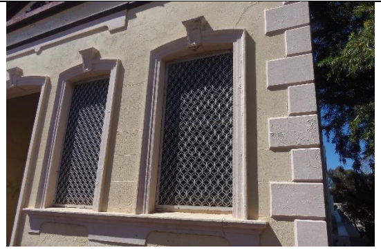
Rendered quoins to corner Source: Stephen Carrick Architects September 2021
