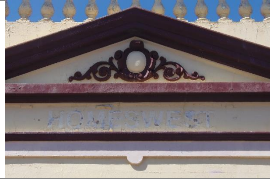
Decorative pediment with "Homeswest" inscribed below Source: Stephen Carrick Architects September 2021
