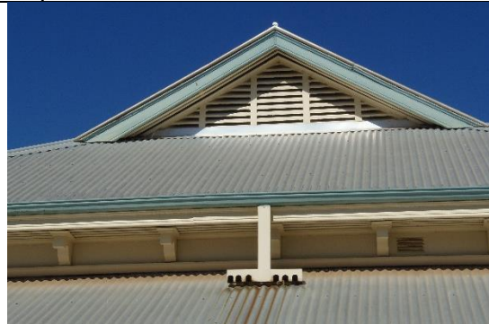
Ventillation gablet Source: Stephen Carrick Architects September 2021
