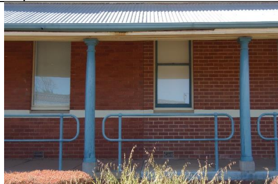
Railing to front verandah Source: Stephen Carrick Architects September 2021
