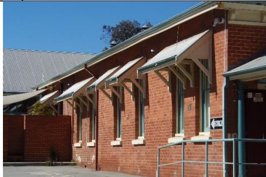
East awnings to central building Source: Stephen Carrick Architects September 2021
