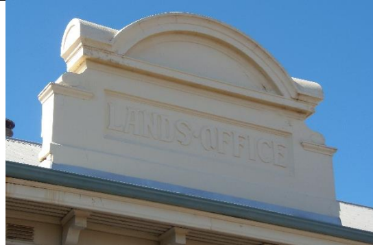
Signage Pediment 'Lands Office' Source: Stephen Carrick Architects September 2021
