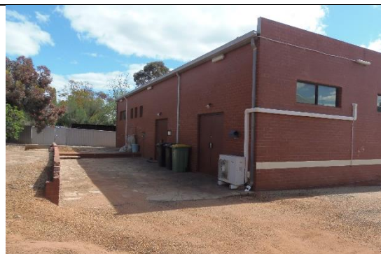
Rear of building Source: Stephen Carrick Architects October 2021
