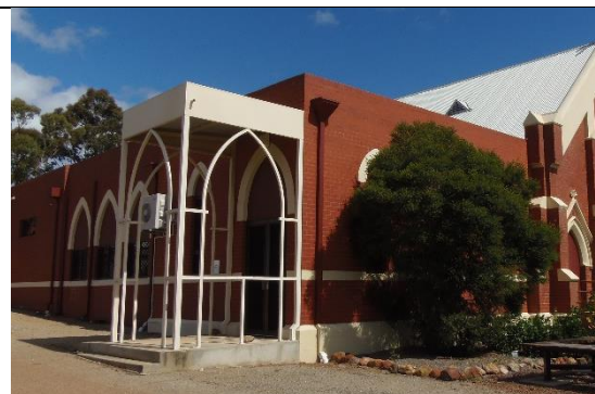
Entrance to northern corner Source: Stephen Carrick Architects October 2021
