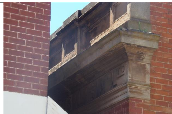
Parapet to rear building Source: Stephen Carrick Architects September 2021
