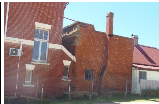
1895 structure attached to the rear Source: Stephen Carrick Architects September 2021
