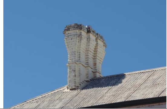
Chimney Source: Stephen Carrick Architects September 2021
