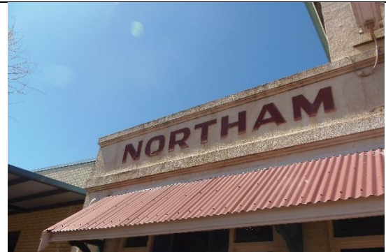
Northam sign Source: Stephen Carrick Architects September 2021
