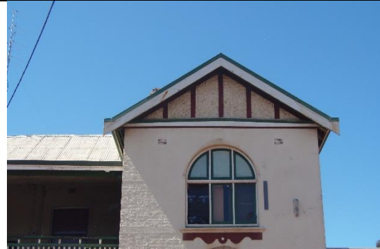
Gable end of southern projecting wing Source: Stephen Carrick Architects September 2021
