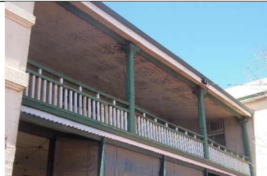
Central two storey verandah Source: Stephen Carrick Architects September 2021
