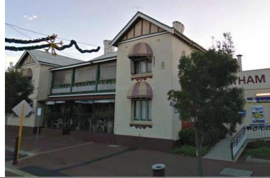
West Façade Source: Municipal Heritage Inventory, 2012
