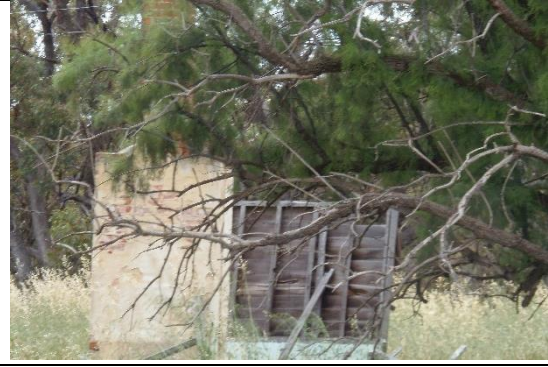
Associated structure Source: Stephen Carrick Architects October 2021
