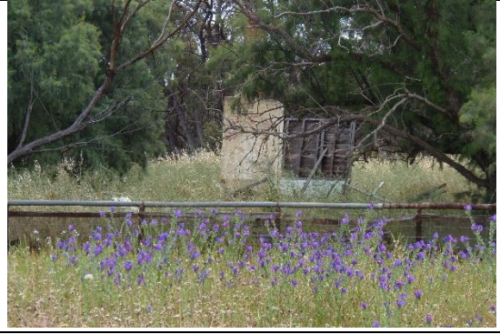
Associated structure Source: Stephen Carrick Architects October 2021
