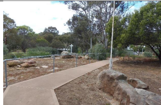
Concrete pathway Source: Stephen Carrick Architects October 2021
