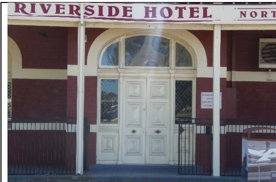
Ground Floor entryway Source: Stephen Carrick Architects September 2021
