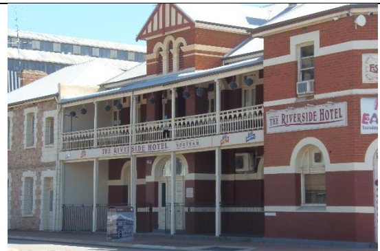
Verandah to south facade Source: Stephen Carrick Architects September 2021
