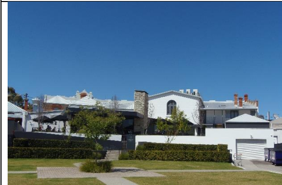
Contemporary addition to the rear Source: Stephen Carrick Architects September 2021
