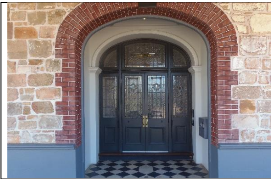
Ground Floor entry Source: Stephen Carrick Architects September 2021
