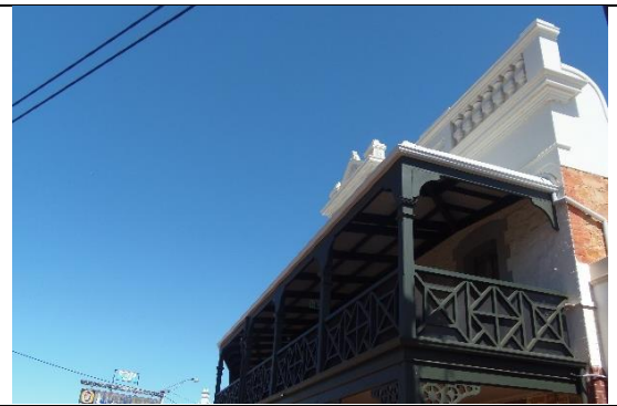
Verandah to front facade Source: Stephen Carrick Architects September 2021
