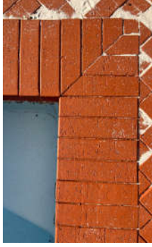
Unit paver header to back of kerb: Midland Heavy Duty Red, laid on edge
