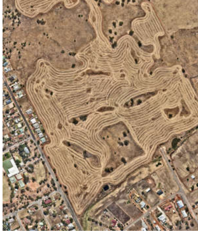
Directional nature of concrete banding takes inspiration from harvesting tracks
