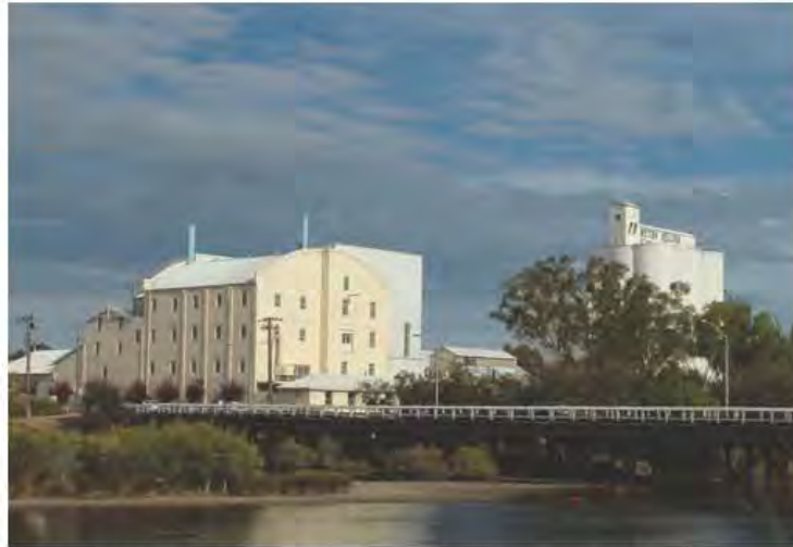
Figure 14. Weston Milling Silos on Fitzgerald Street – the opportunity for an iconic art mural and entry statement into town. (Source: Miiigoria.net)
