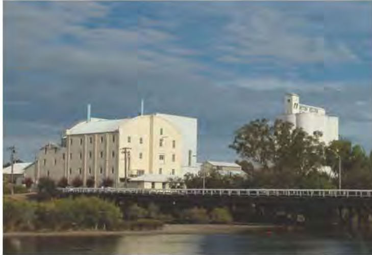
Figure 14. Weston Milling Silos on Fitzgerald Street – the opportunity for an iconic art mural and entry statement into town. (Source: Miiigorn.net)
