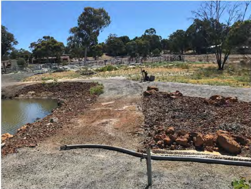
Spillway of Dam
