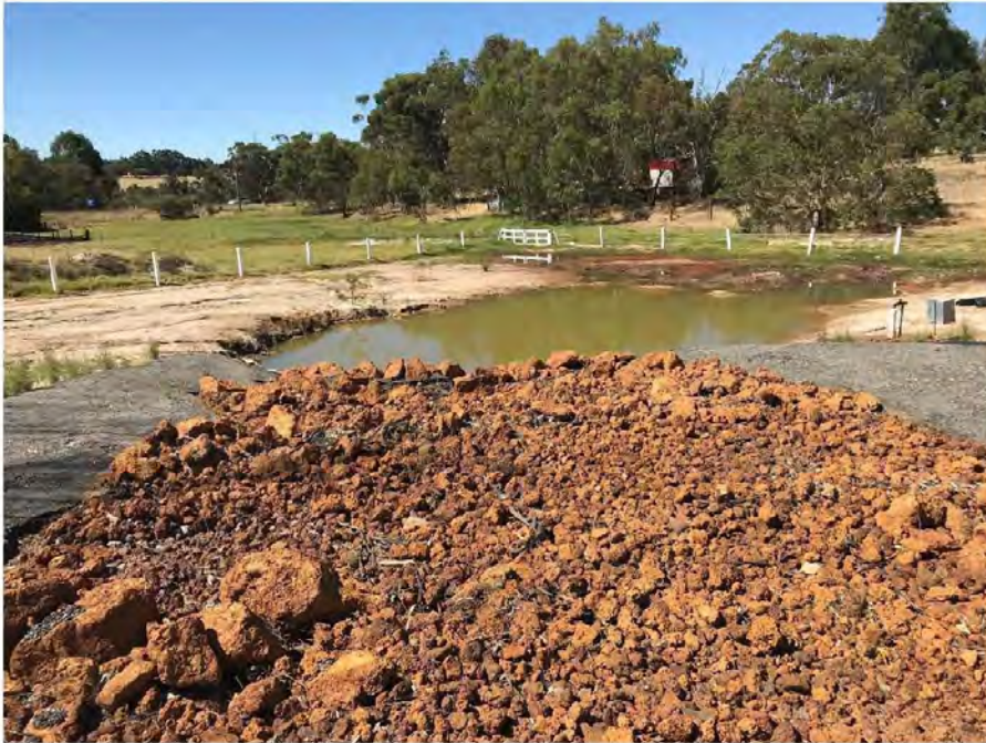
View of spillway and stilling pond to the north
