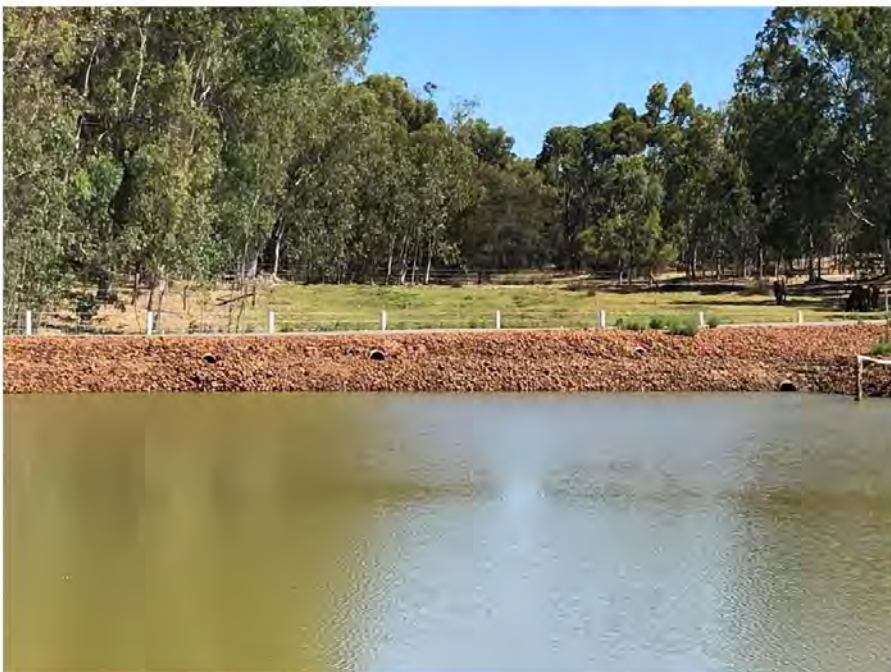
View of driveway and culverts
