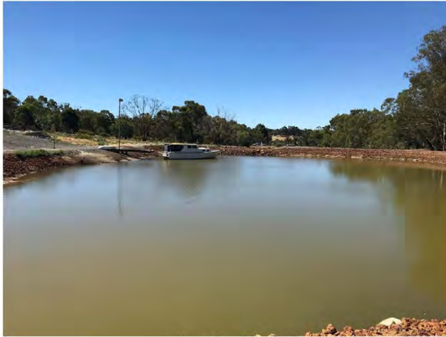
View of Dam Looking North
