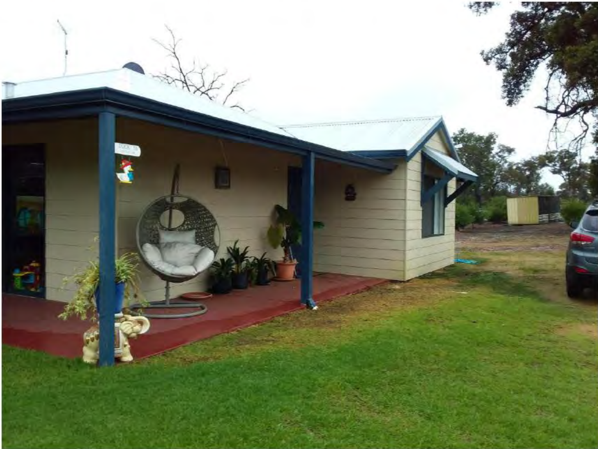
Photo of Main Residence – Lot 363 Glenmore Drive, Bakers Hill
