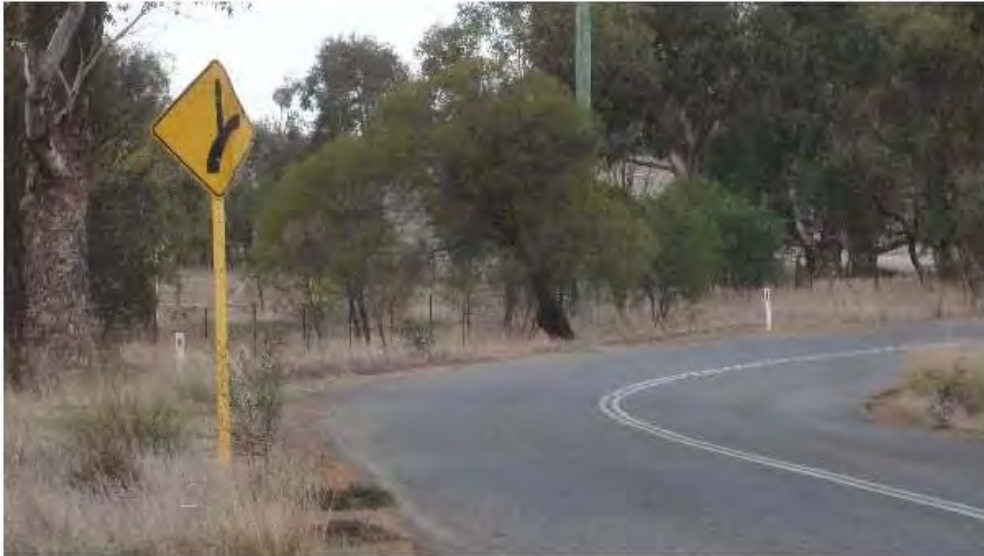
Finding 2.12 – Damage to warning sign
