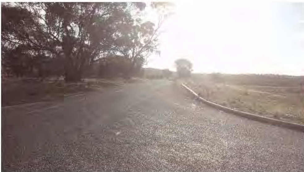
Finding 2.15 – Intersection sight distance – Example of poor SISD (note sun glare in sunset conditions)
