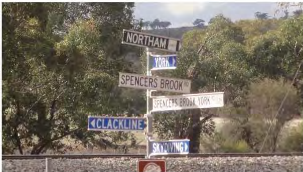
Finding 2.22 – Spencers Brook York Road Intersection Signs
