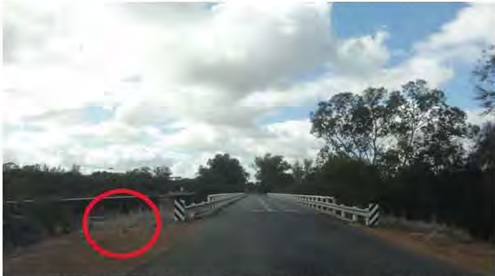
Finding 2.14 – Bridges – Barrier system length would not provide protection of errant vehicle
