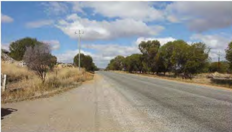
Finding 2.4 – Quarry Access – Sight Distance to the south
