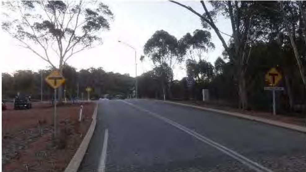
Finding 2.21 – Great Eastern Highway warning signs
