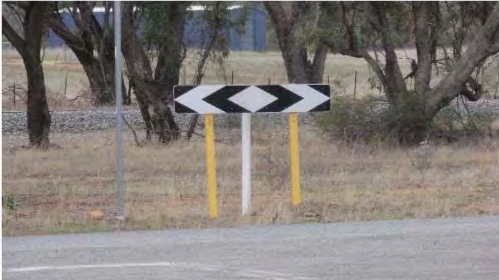
Finding 2.5 – Intersection warning signs –Example of incorrect sign used
