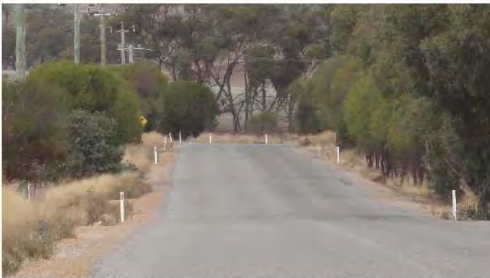
Finding 2.6 – Vegetation Maintenance – Vegetation obstructing warning sign
