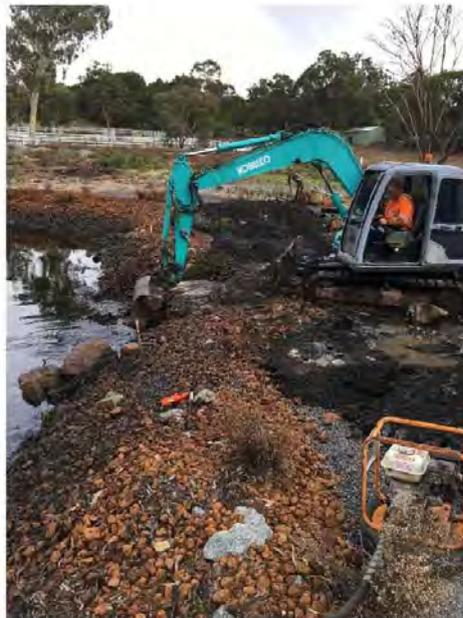
d. Completion of base earthwork level. this is about 600mm lower than the invert level of the upstream culvert
