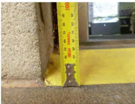
60mm abutment at threshold to enter the Library at the second entrance
