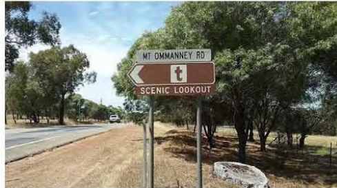
Wrong symbol, should have the lookout symbol (camera), no advance warning signs for this location
