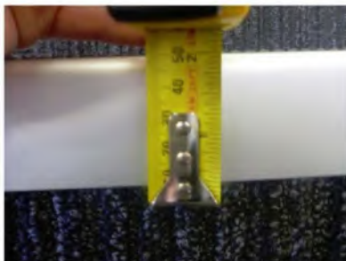
Increased nosing profile (50mm) down riser
