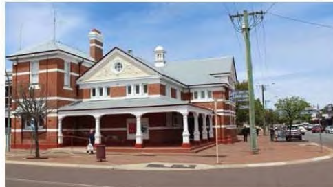
Examples of heritage buildings
