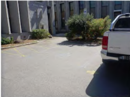
ACROD bay at Fitzgerald St small carpark
