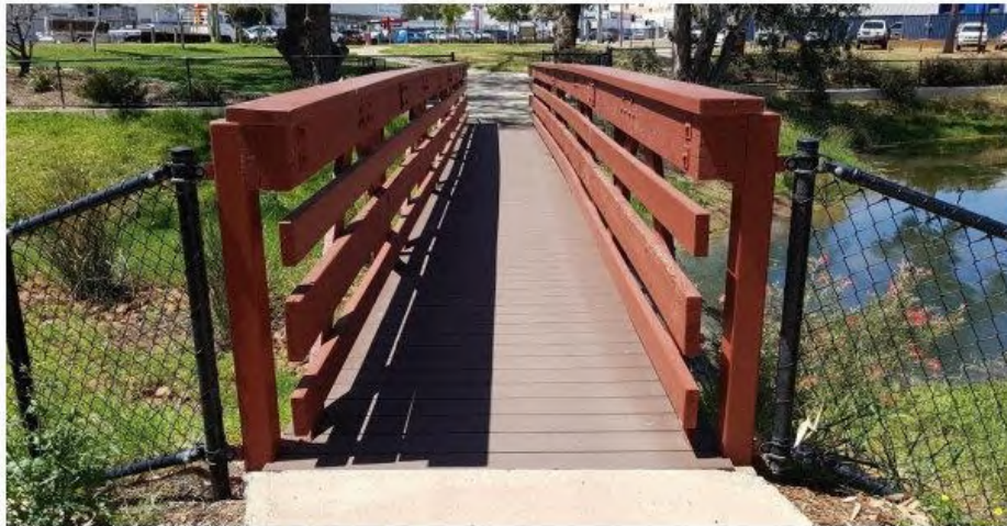
Photo 11: Narrow bridge with bike unfriendly parapets.
