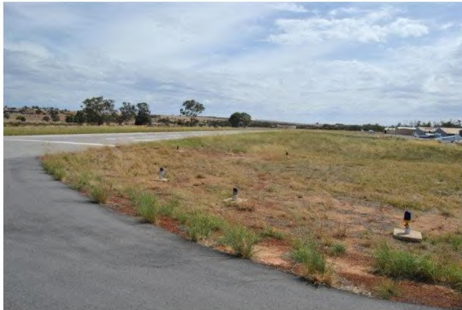
View facing north-west from the southern taxiway. Runway threshold and taxiway edge lighting.
