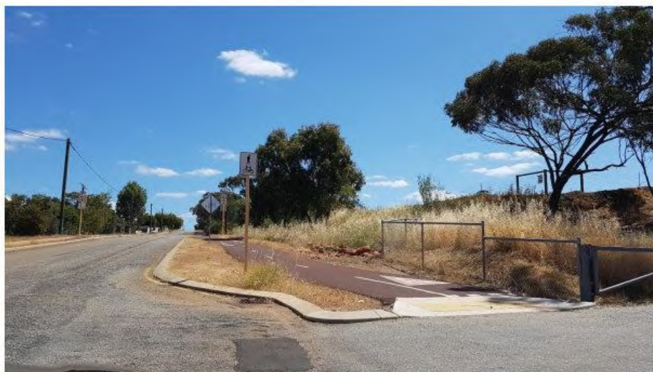
Photo 1: A section of Shared Path with signs and line marking.
