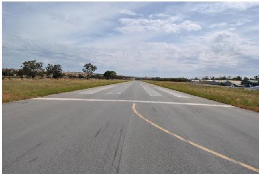
View facing north-west along runway. Faded threshold markings for Runway 32.
