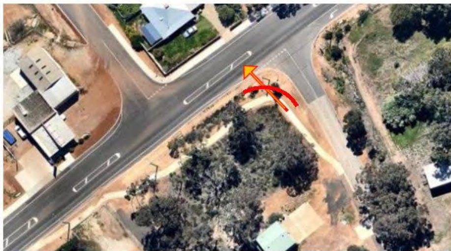
Figure 7.1: A suitable safety barrier may prevent a serious incident.
