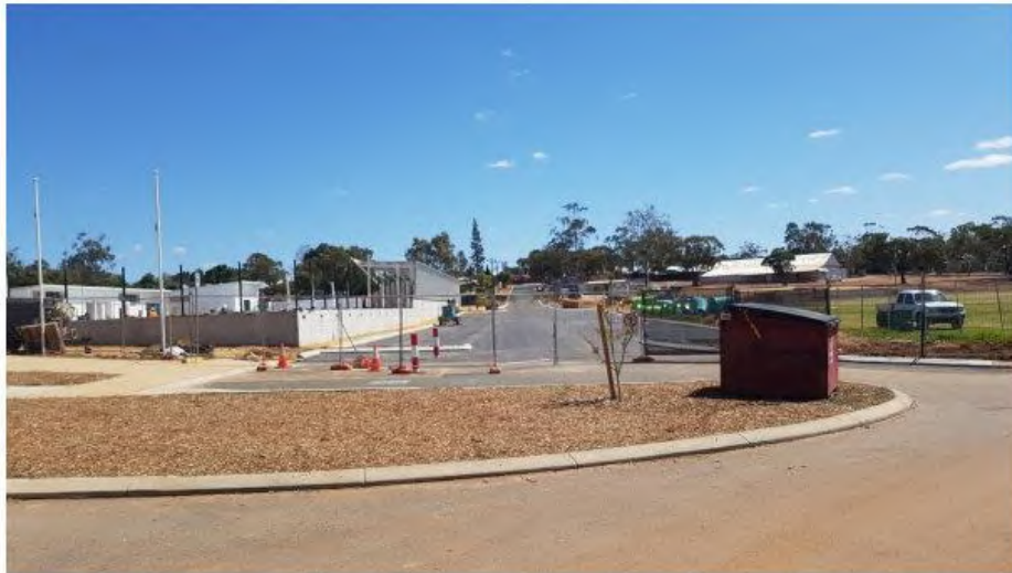
Photo 5: New Northam Aquatic Centre, during construction, adjacent the Recreation Centre.
