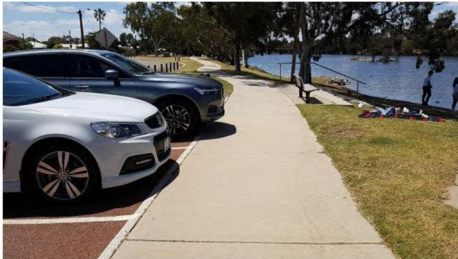
Photo 18: Lack of wheel stops means parked cars become a hazard to path users.
