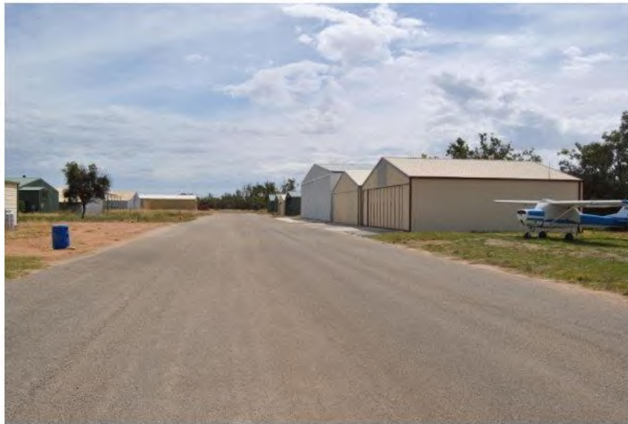
View facing north-west along the line of 7 private hangars behind the main apron.
