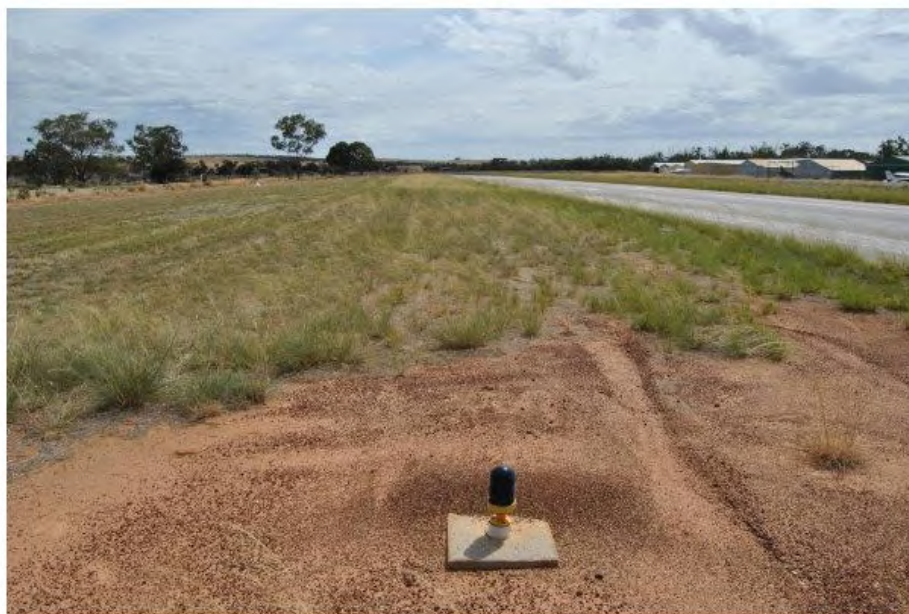
Concrete blocks should be flush with the surrounding area on the Runway Strip.
