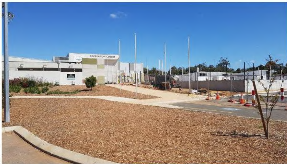
Photo 6: The Northam Recreation Centre and the adjacent Swimming Pool (during construction).
