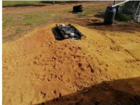
Septic tank fully covered
