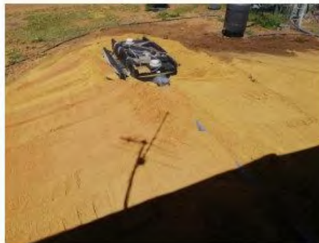
Septic tank showing painted pipes
