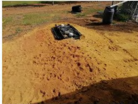
Septic tank fully covered
