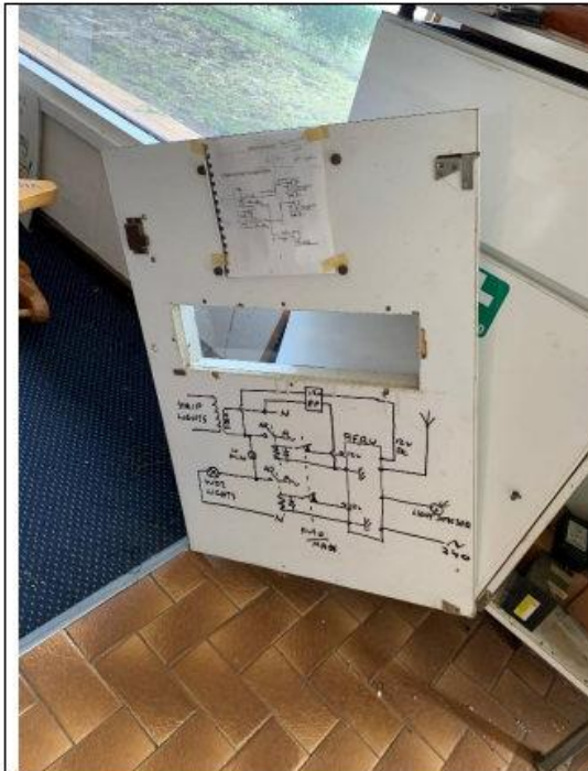
Image 5: Control Panel Door-Circuit Diagram
