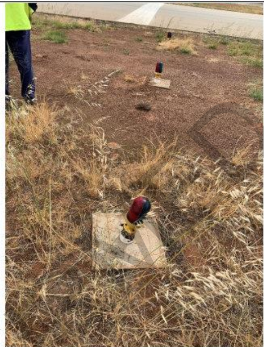
Image 6: Non compliant Threshold/End Pattern
