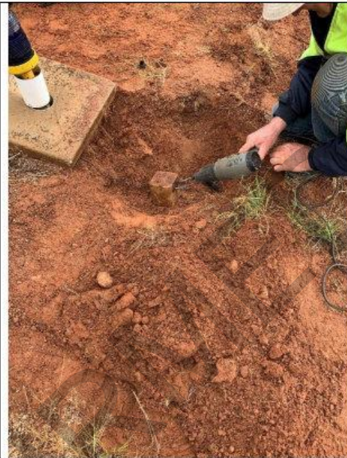
Image 10: Reconnection after Insulation Tests
