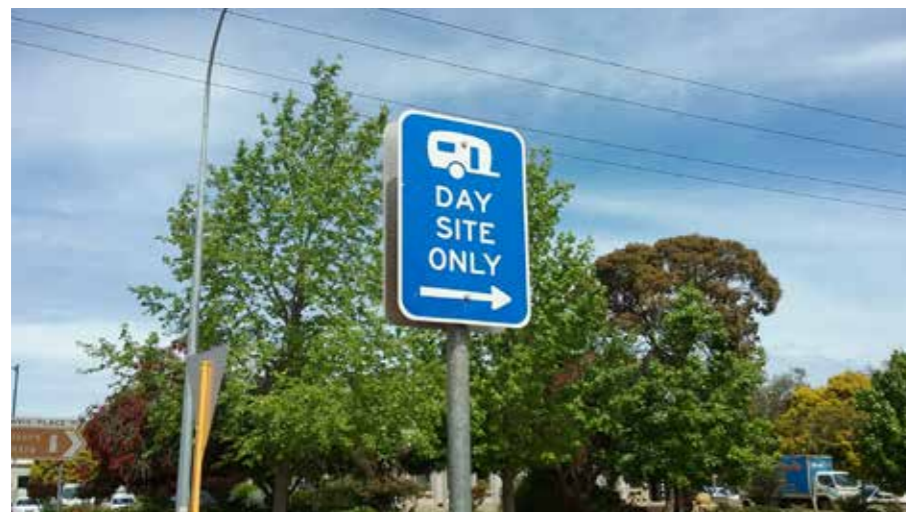
Remove old signage
