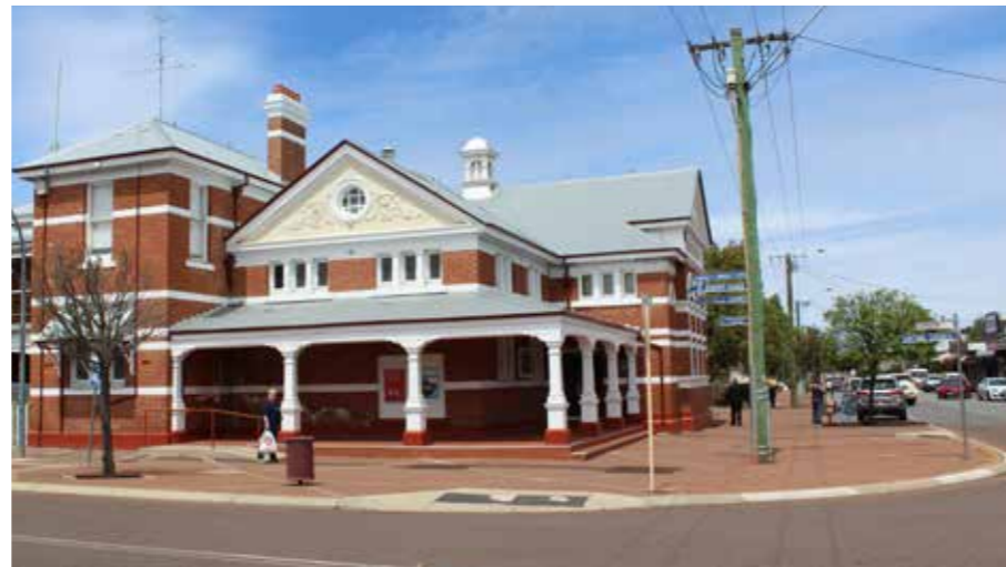
Examples of heritage buildings
