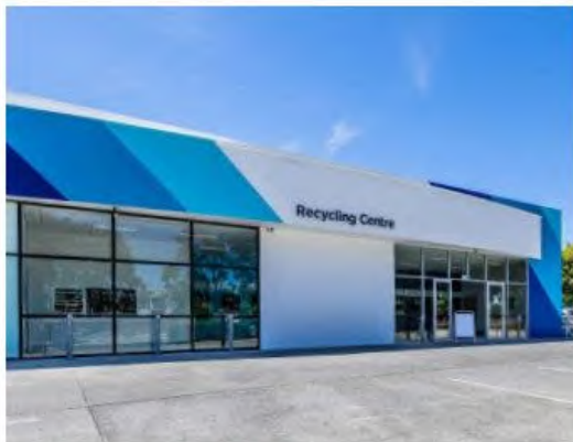
Container deposit recycling centres
