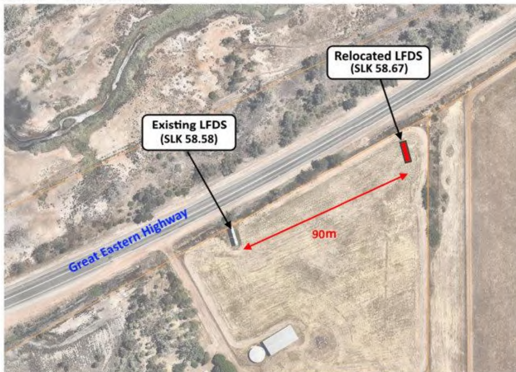
Figure 2-1 Relocated LFDS Position
