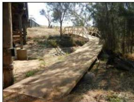
Yilgarn Avenue, Northam – Path appears to just end on approach to bridge over Mortlock River. Users may cross on the vehicle bridge, unaware that a separate bridge has been provided for them.
