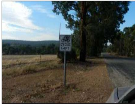
Hawke Avenue, Wundowie – Regulatory signage has been installed but the cycling infrastructure is not clearly defined (e.g. through linemarking or coloured paint)
