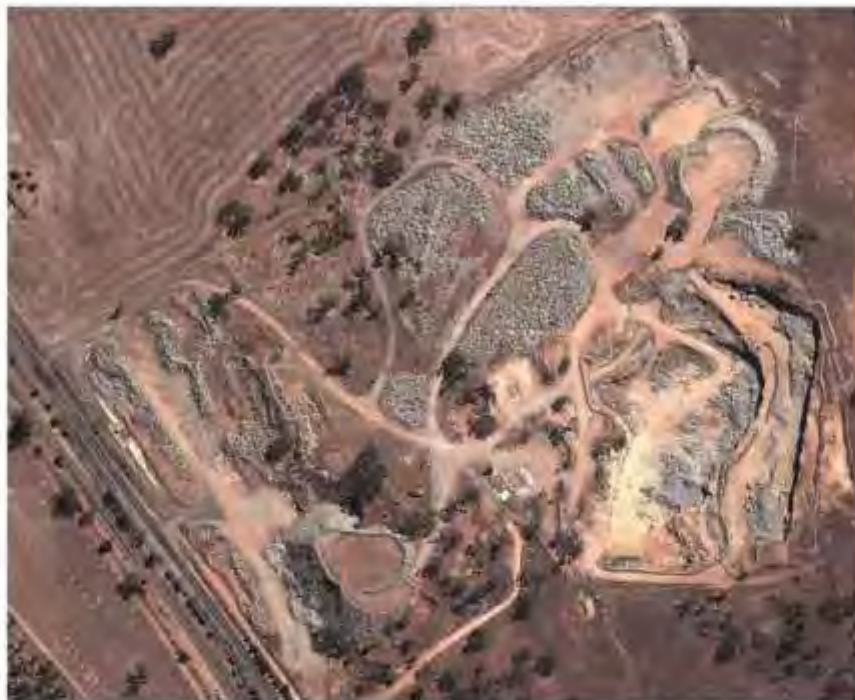
Figure 1: Overview of Site
