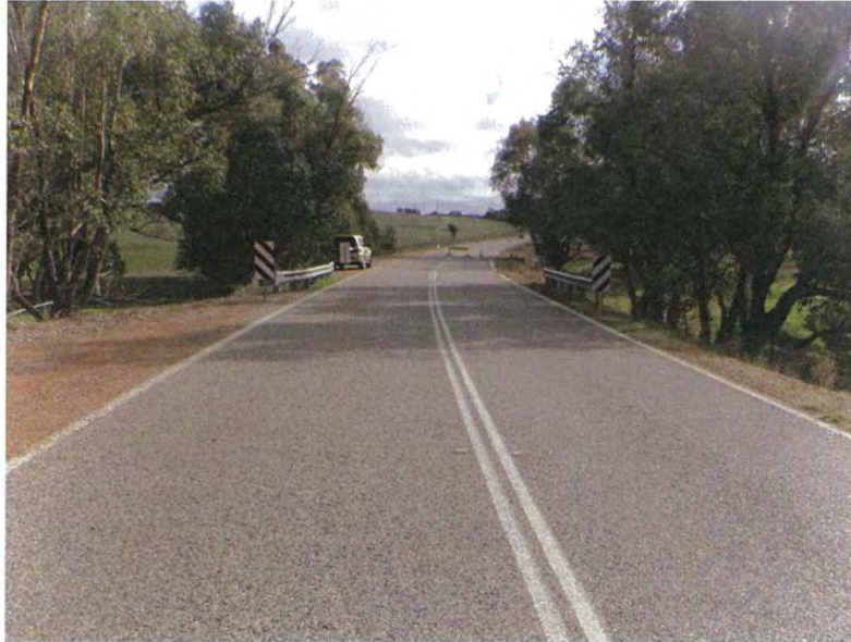
Photograph 1: Top of bridge from Approach 1.
