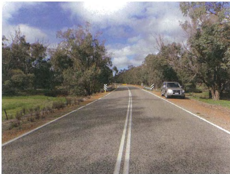
Photograph 2: Top of bridge from Approach 2.
