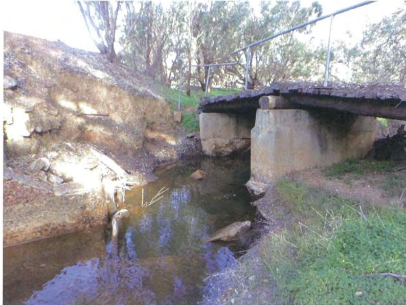
Photograph 13: Pedestrian bridge to left hand side of Bridge 5029.
