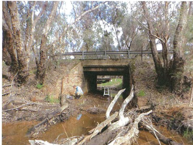
Photograph 4: Right Hand Side of Bridge.
