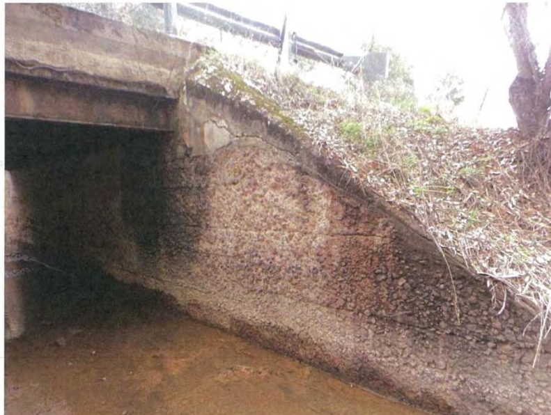
Photograph 6: Typical abutment (Abutment 2).
